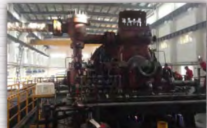
NH3 Refrigeration Compressors (LP/HP) c/w Mechanical Drive Steam Turbine
