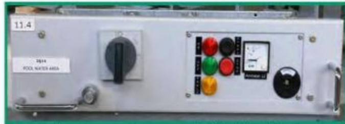
Maloperation protection prevent travel of the withdrawable-units when the master switch is "ON"
