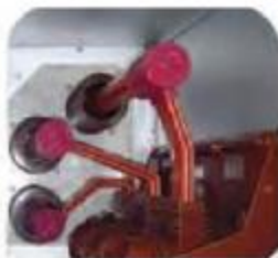
Busbar compartment of RG-MEE
