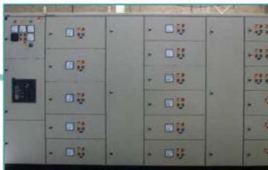
Low Voltage Switchgear Fix , Free Standing—Modular Tech. RG-BerliAnt Type
