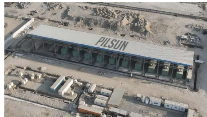
Packaging | Jask power plant
